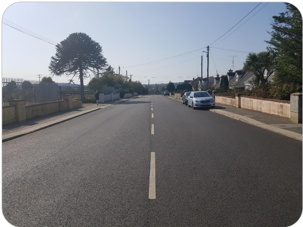
Figure 7 – Clonattin Road (view to south-west from junction with Clonattin Village access road)
